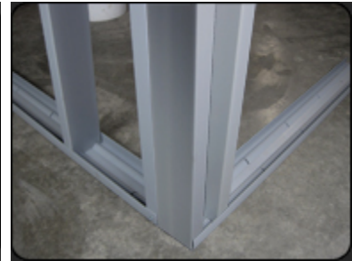
Install the next stud flush with the end of the first track to create the outside corner, screw this stud to the one next to it for added strength
