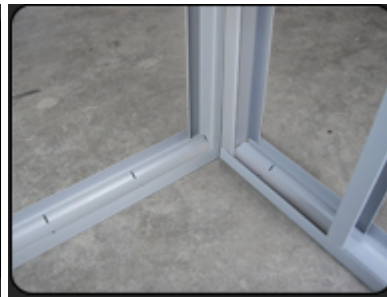
Install the corner stud into the first slot of the track
