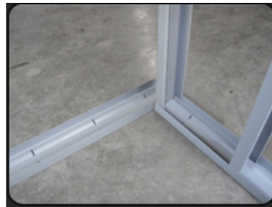
Add the next track to create the inside corner
