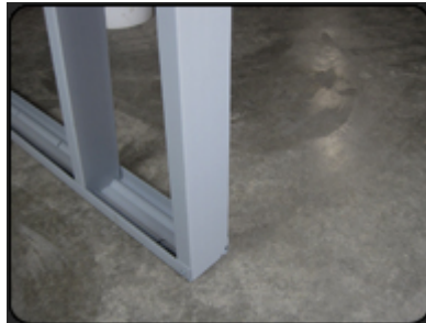
Assemble a wall with the end stud flush with the end of the track
