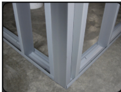
Finish the wall by locking the studs
