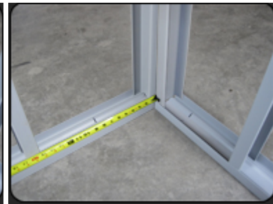
Position the track so the middle of the second stud is 16" from the adjacent wall
