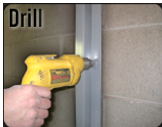
Glue and screw every 18": 3/16" x 1 1/4" masonry screws and OSI QB300 or equivalent
