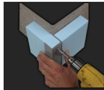
Attach corner bead as seen in the step below
