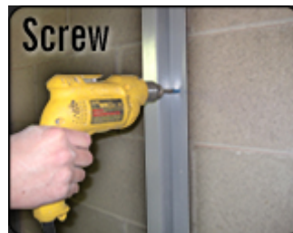
Glue and screw every 18": 3/16" x 1 1/4" masonry screws and OSI QB300 or equivalent
