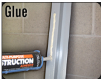
Glue and screw every 18": 3/16" x 1 1/4" masonry screws and OSI QB300 or equivalent
