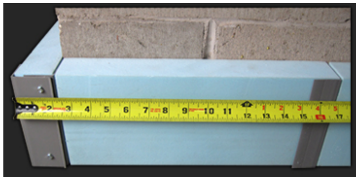
Start on a corner and work away from it. Install the first EcoStud so the center lands at 16" as shown
